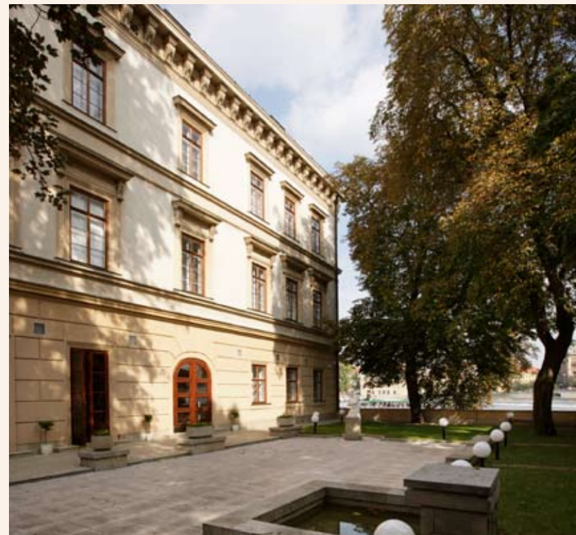
The atrium in front of the southern facade
