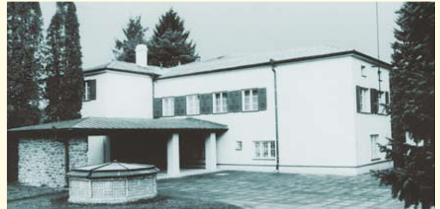
The villa's southeastern façade after refurbishment, 1990
